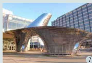
Roof Like Fluid Flung Over the Plaza, 2003 Cannon Center for the Performing Arts N. Front St at Poplar Ave
