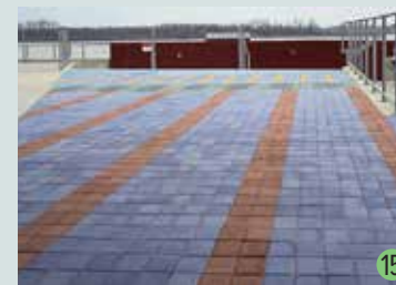
Walkway Paving, 2014 Beale St Landing 251 Riverside Dr
